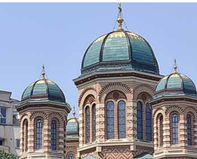
Domnița Bălașa Church, Bucharest KME 'TECU@ Patina Oslo' copper sheets and KME Natural copper rain gutter system
