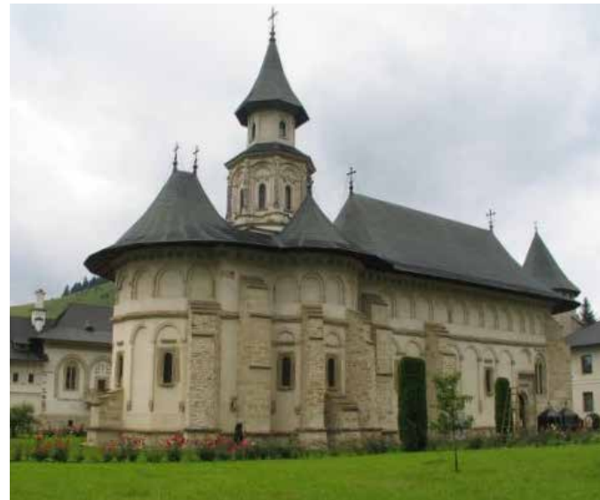
Dragomirna Monastery, Suceava / KME Natural copper sheets
